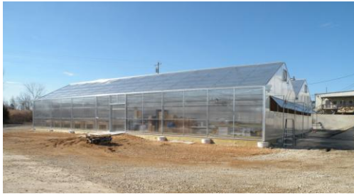
Lake Area Industries Greenhouse N Business Rt 5
